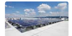
Solar panel installation
