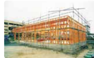
A Ministop store under construction
