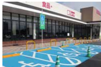
Parking lot guardrails
